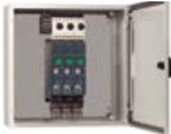
Several ATV320B drives with GV2 circuit breakers directly mounted
